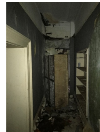
4. Ground floor corridor
