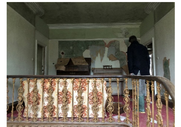
5. Landing above the main hall stairs
